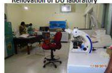
Renovation of DU laboratory
