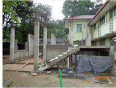
Construction of changing rooms for student at NTS
