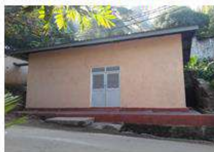
Construction of generator room
