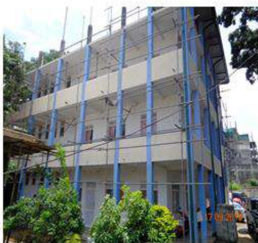
Construction of nurses quarters stage 3
