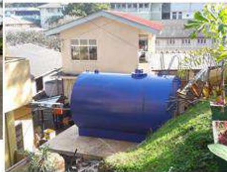
Construction of new diesel tank for laundry
