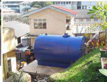
Construction of new diesel tank for laundry
