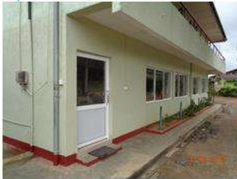
Renovation of demonstration room at NTS
