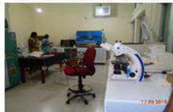
Renovation of DU laboratory
