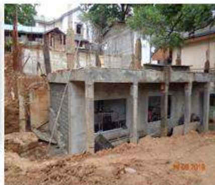
Construction of antibiotic drug stores- stage 2
