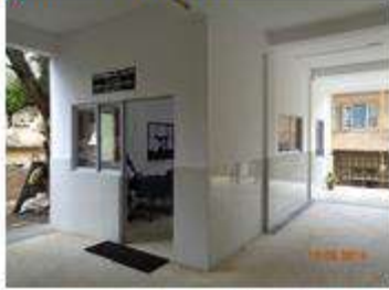
Construction of SGNOs, office at DU & wash room at ward 23
