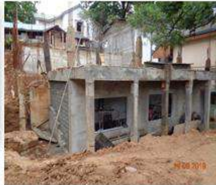
Construction of antibiotic drug stores - stage 2
