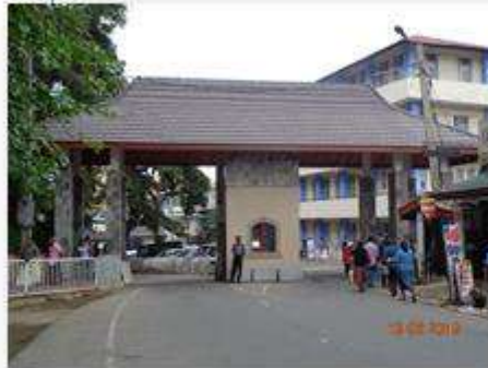
Construction of hospital entrance from Hanthana area
