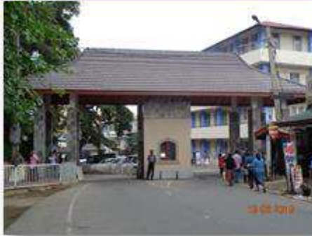
Construction of hospital entrance from Hanthana area
