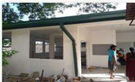
Construction of antibiotic drug stores stage 1 (balance work)
