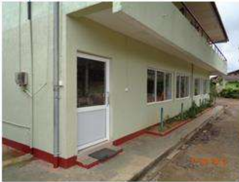
Renovation of demonstration room at NTS
