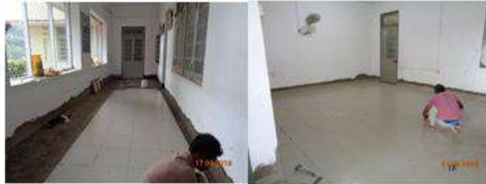
Renovation of main building ground floor at NTS
